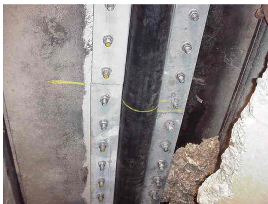
Fig 10.11.12 Omegaprofiel na montage
