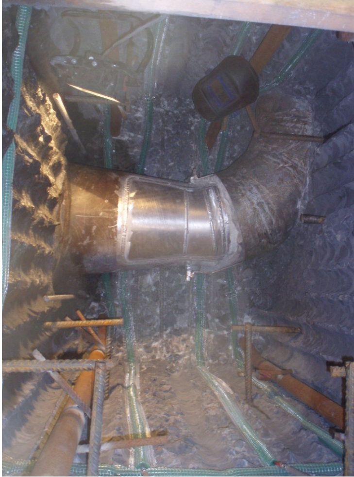
Figuur I.4: Mock-up: na reparatie reducer.
