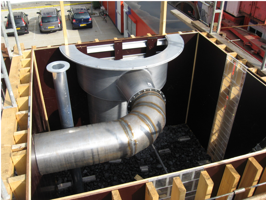
FIG. 3: Mock-up of reducer prior to pouring concrete.
