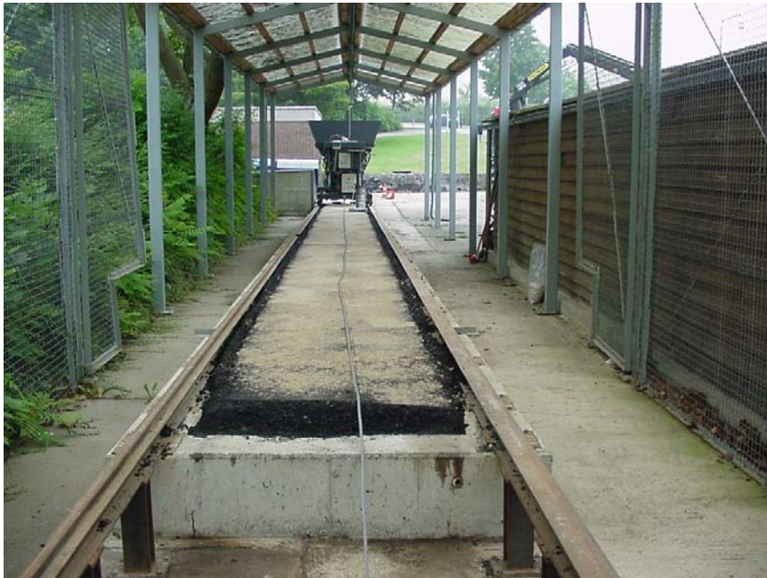
Figure 2: The material was applied using an asphalt spreader for cycle paths.
