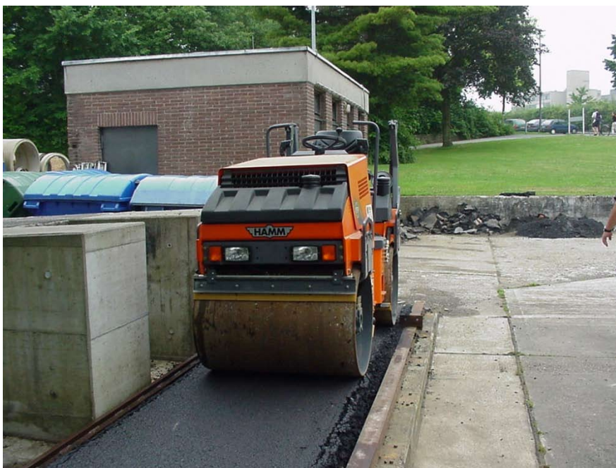
Figure 3: The compacting was performed using a HAMM vibrating roller
