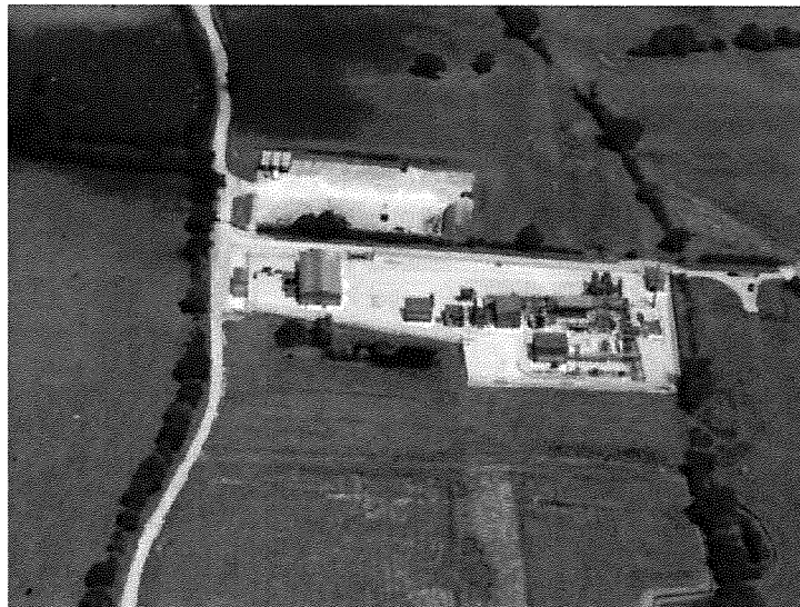
Figure 5. Hole House facilities
