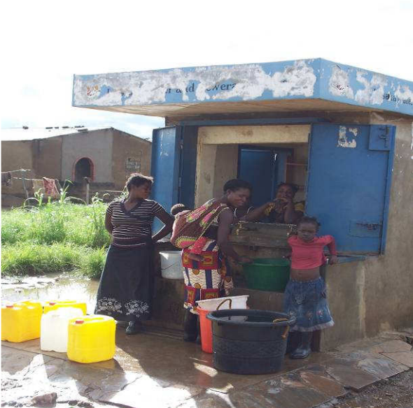
DTF sponsored water kiosk
