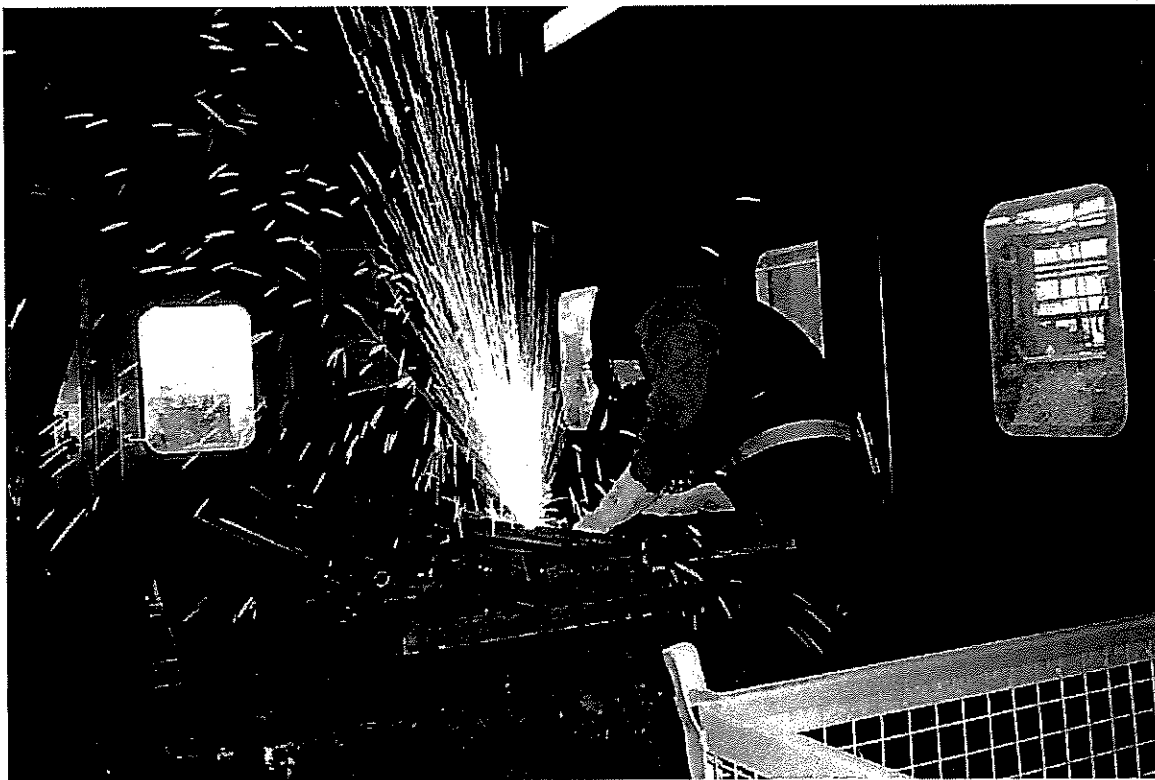
Figure 7-8: Thermal cutting (Picture by courtesy of EWN)
