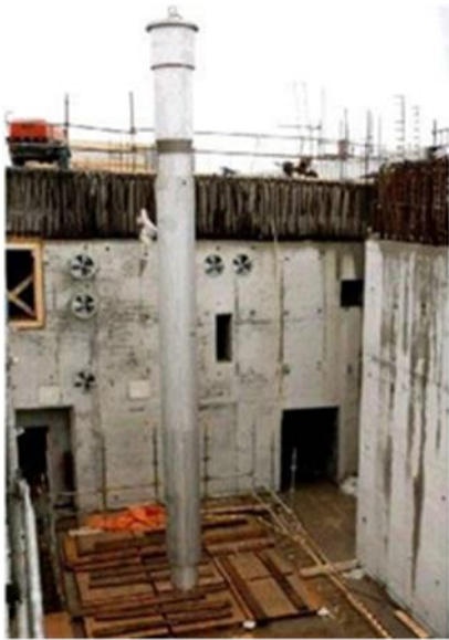
Figure A.4 Emplacement of wells during construction
