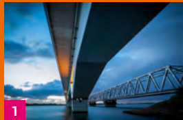
1 High-speed railway and railway bridge crossing the Hollandsch Diep, with the Hoeksche Waard and the Island of Dordrecht on the opposite side. (p 1)
