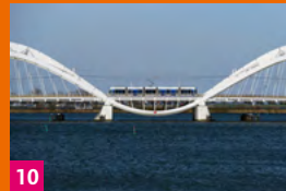
10 The Enneus Heerma bridge connecting Zeeburger island with Steiger island, gateway to IJburg. (p 20)
