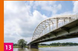
13 The Wilhelmina bridge over the IJssel, at Deventer. (p 28)
