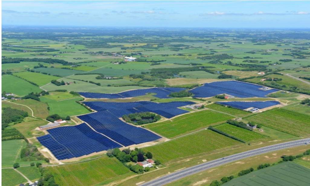
Figure 5.3 - Sejling Hede sun heat plant for district heating developed and owned by Silkeborg utility
