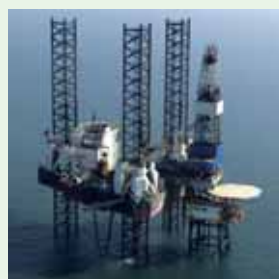
In 7 months Wintershall dismantled the K10 V platform and after refurbishment installed the L5C platform for the extraction of approx. 4.3 bln m 3 of Natural gas. The reuse of a platform can both be environmental friendly and economical.
