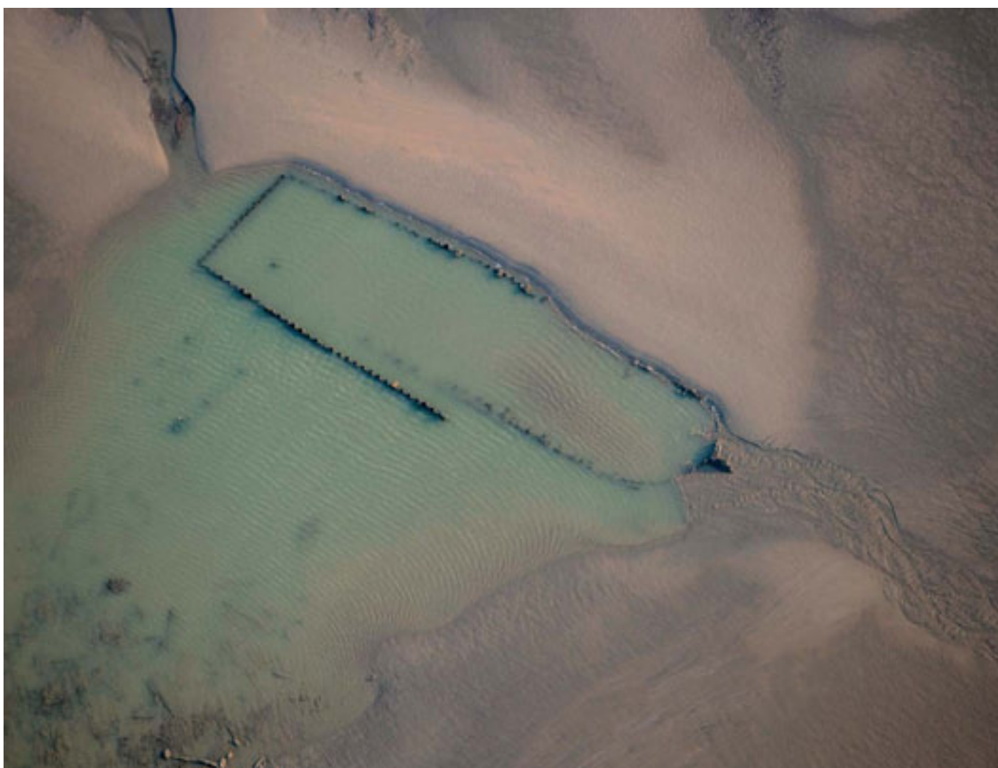
FIGURE 2: The site of the Dutch East Indiaman Amsterdam protected by a sheet piling. PHOTO: ENGLISH HERITAGE
