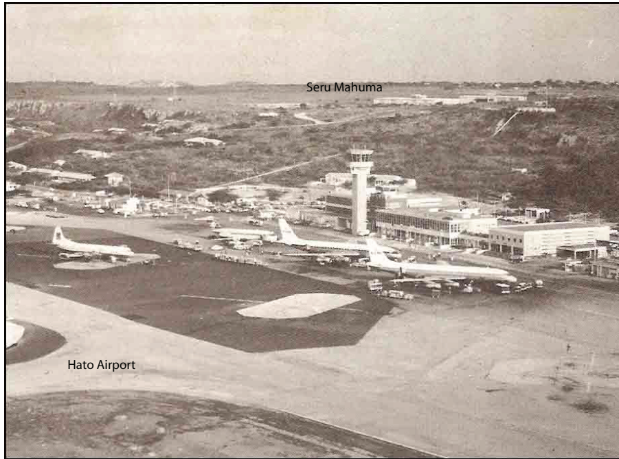
Fig. 4: The Dr. Plesmann (Hato) airport, with in the background on the hilltops the building of the Department of aviation, c.q. the location of the meteorological observatory from 1976 and forth.
