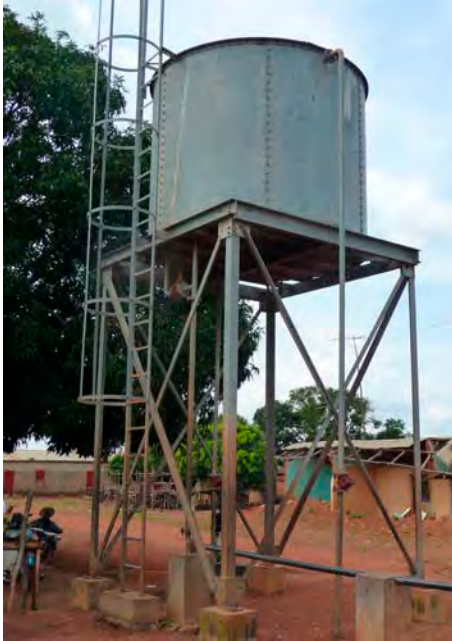
Small piped water supply system
